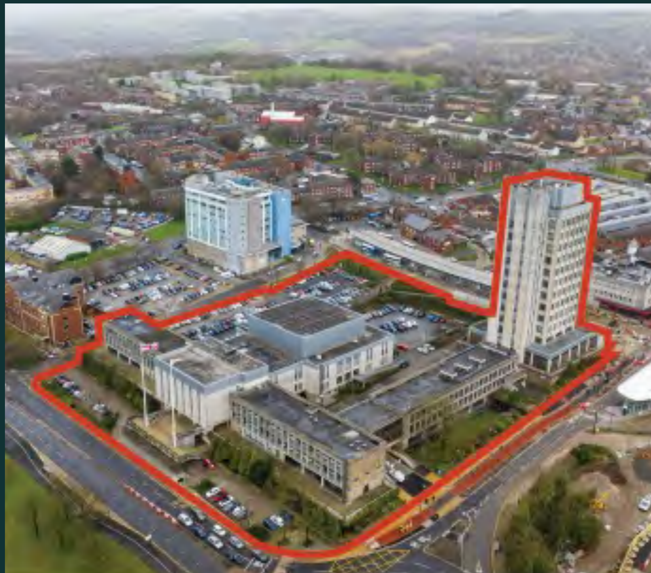
→ FIG. C3 – AERIAL VIEW OF THE CIVIC CENTRE AND QUEEN ELIZABETH HALL
